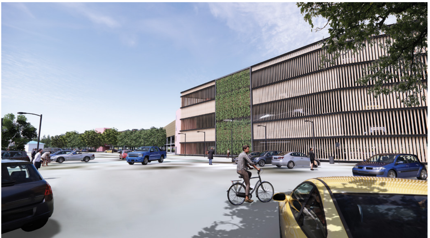
Front view of the extension to the multi-storey car park
