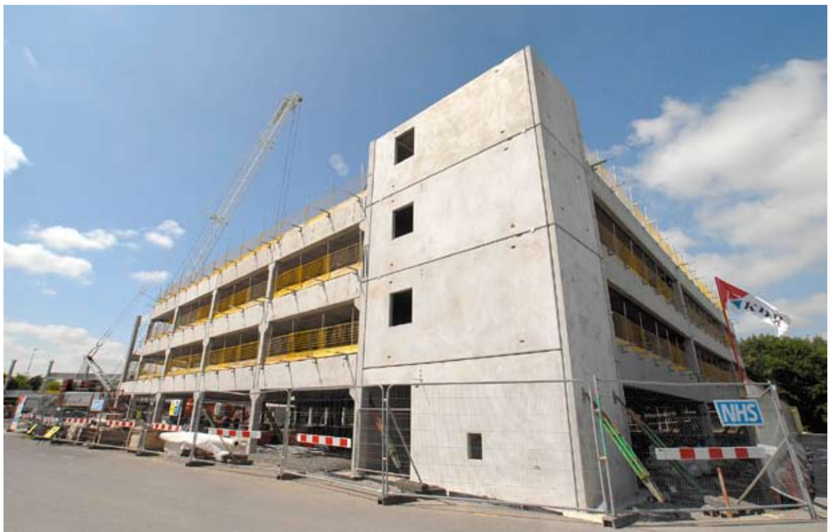
New multi-storey car park on target for completion in December 2009
