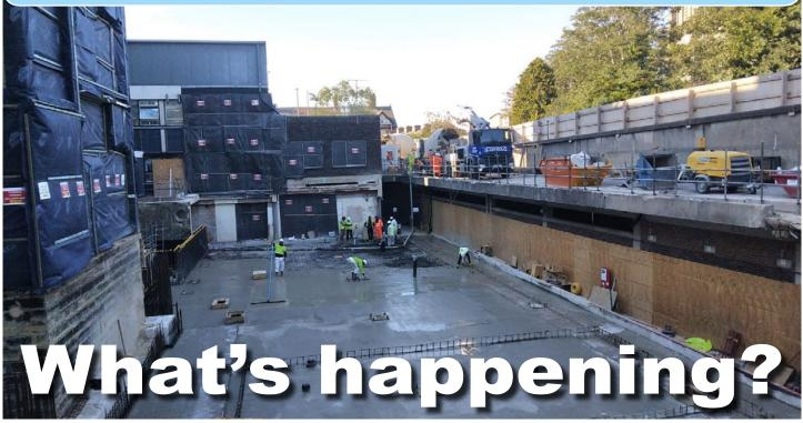
Now that the crane is in place, preparations for the concrete foundations and basement floor are well underway. The concrete slab is being created with responsibly sourced steel rebar rods that are formed from 90% recycled materials. The rods vary in diameter and shape some are up to 2.5cms, and are secured with wire ties and all tied by hand. This is a labour-intensive task for our team of steel fixers.
